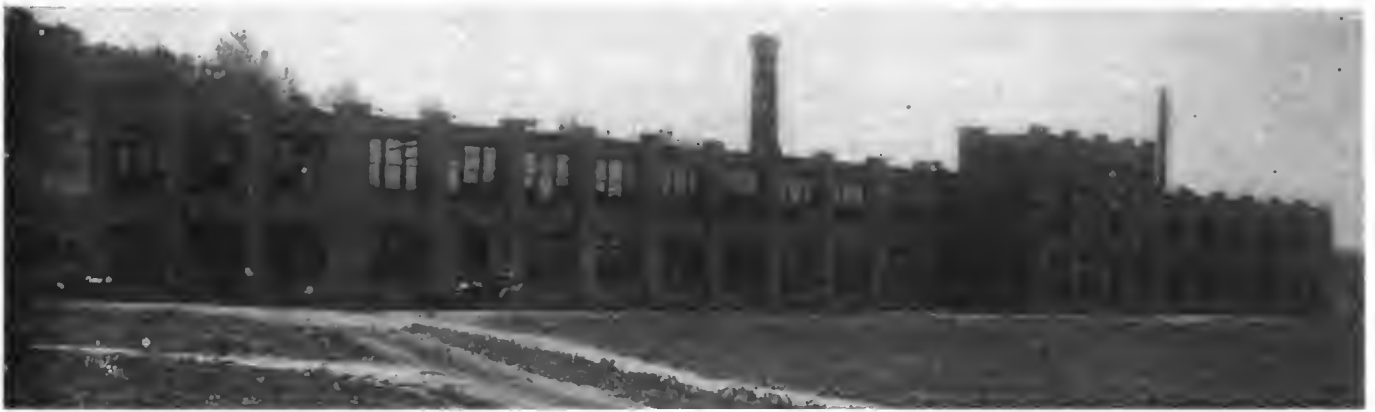
Spaciousness Shown in General View of the Plant of the Mora Motor Car Company, at Newark, New York
